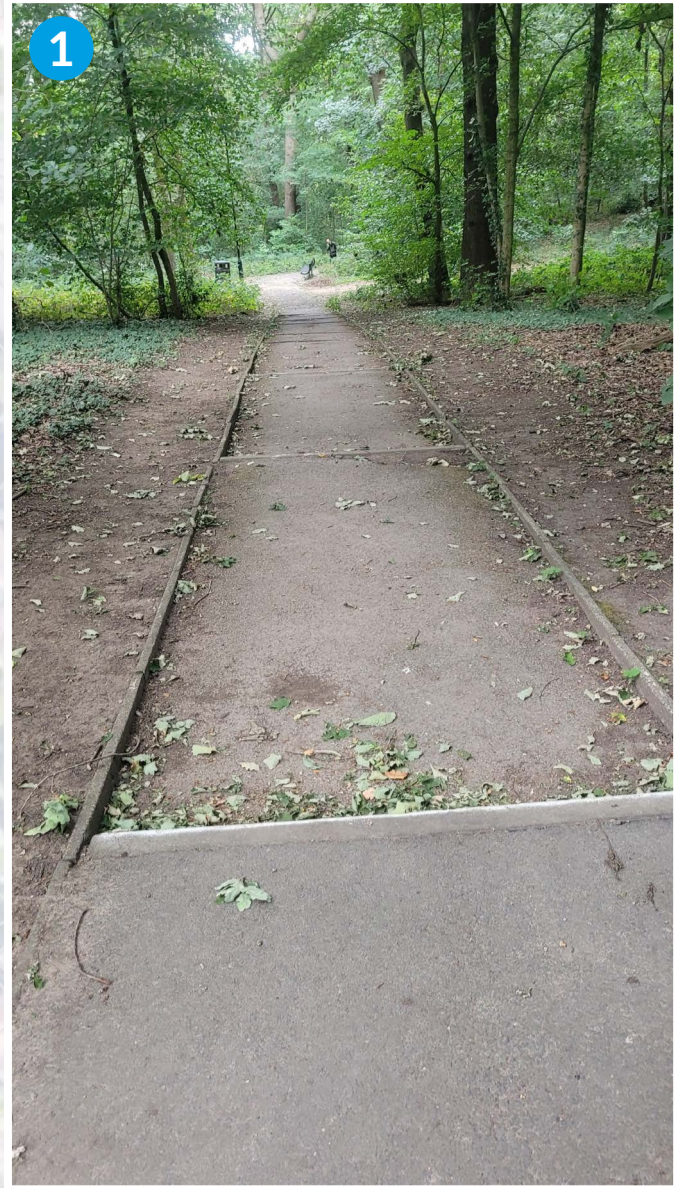
Existing bitmac stepped ramp in reasonable condition.
