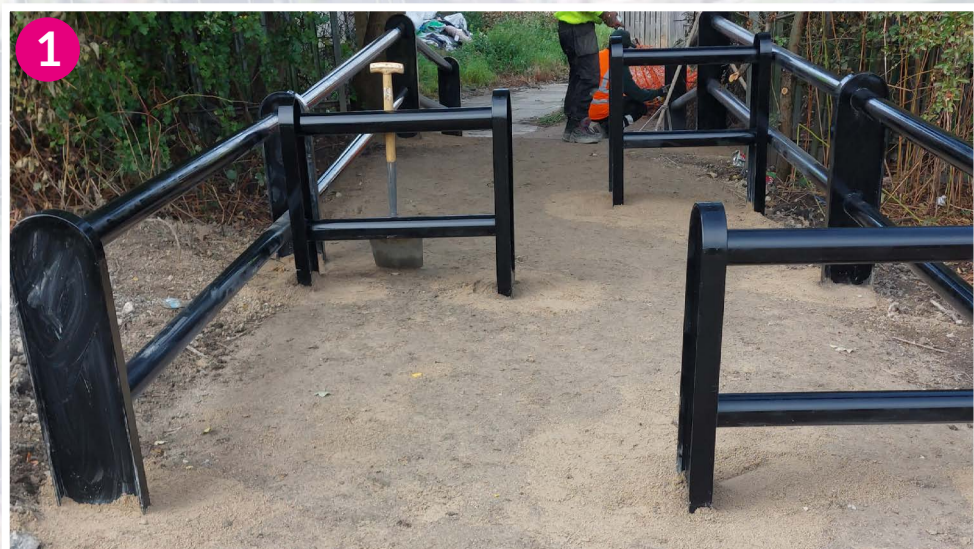
Chicanes to be placed at entrances and to replace some bollards to prevent/slow down quad bikes and dirt bikes.
